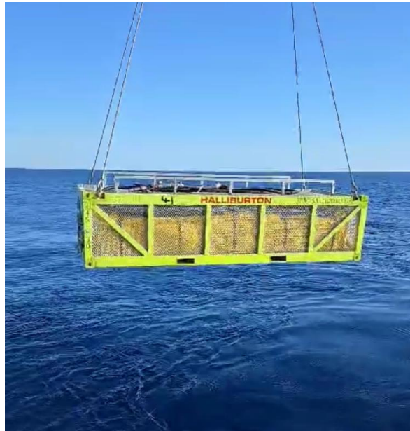
Figure 4: Subsea TEG Storage Basket Deployment
