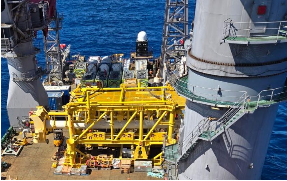
Figure 7: 42" Subsea PLR on deck
