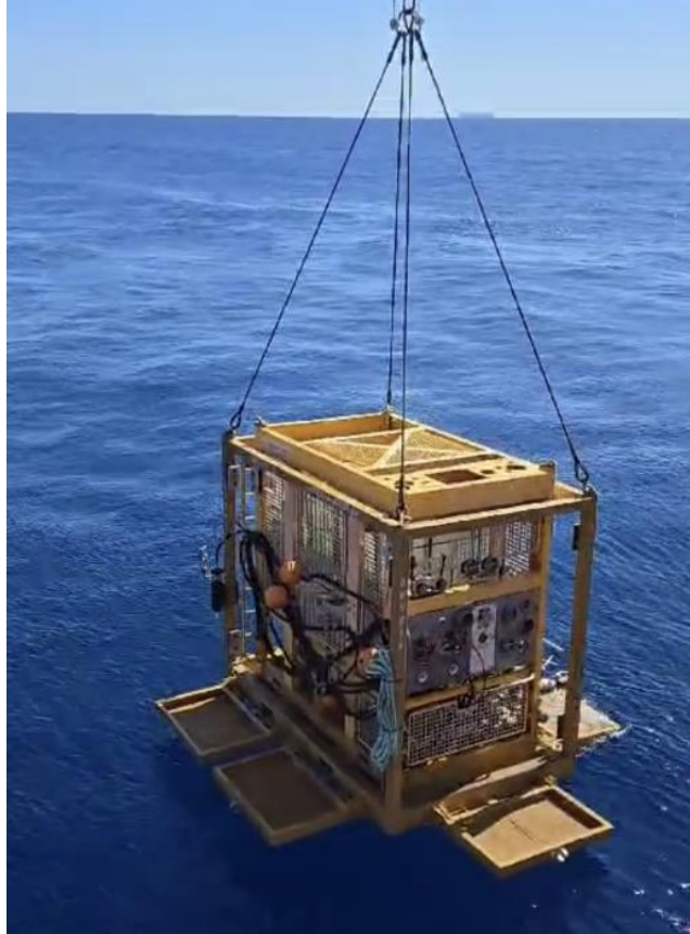
Figure 3: Subsea Pump Unit Deployment
