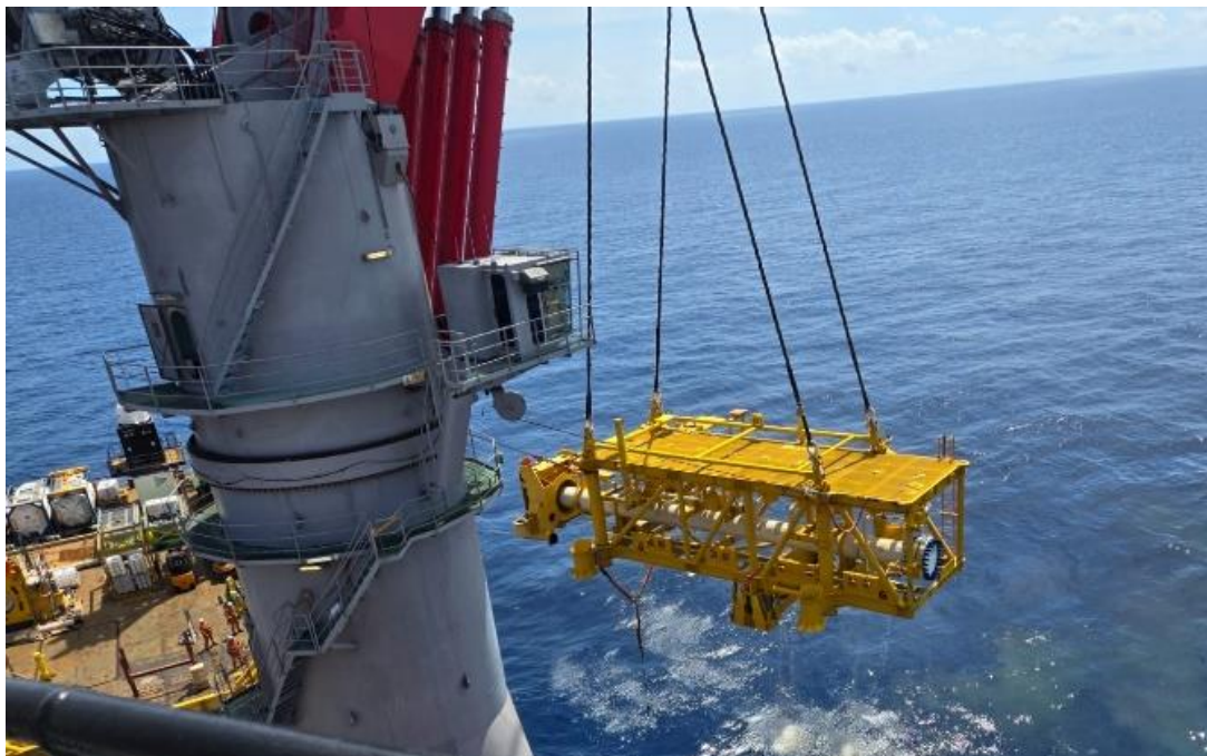
Figure 8: Deployment of 42" PLR
